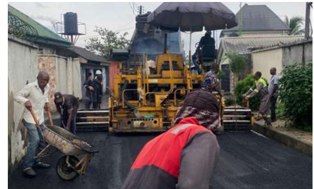
Work going on to expand and asphalt a community road © IPL Nigeria
