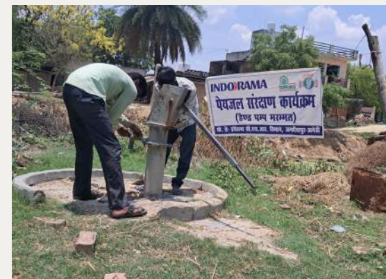
Two new hand pumps were installed, and 17 existing hand pumps were repaired in nearby villages around the factory in Jagdishpur. © IJ India
